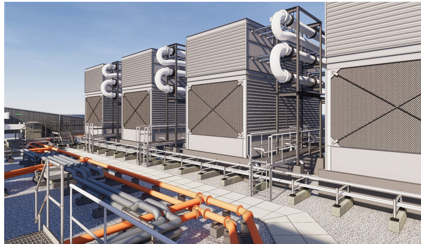
Modular roof installation
